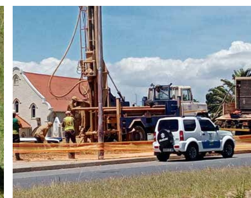
Fig. 4.100. Borehole Drilling at Target A (CCT, 2021)
