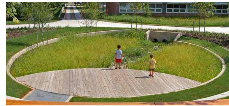
Fig. 4.107. Sustainable urban drainage retention pond,
