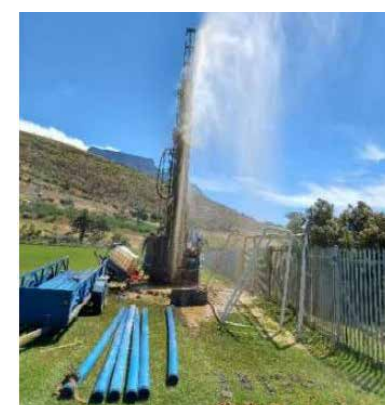
Fig. 4.101. Borehole Drilling at Target B (HHO, 2022)
