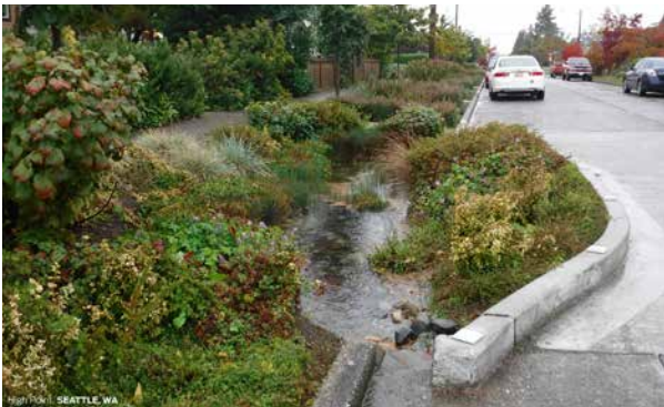
Fig. 4.111. SUDS storm water road bump-out and swale for planting and detention
